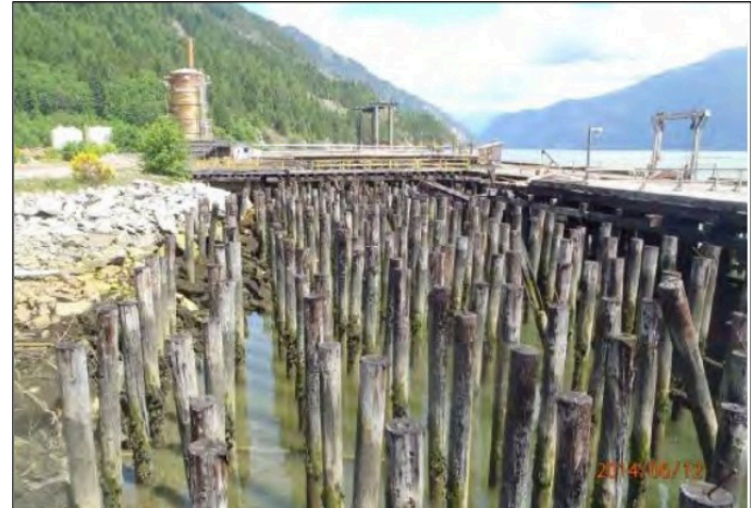
Old marine infrastructure that was removed during restoration Photo by: Keystone Environmental Consultants
