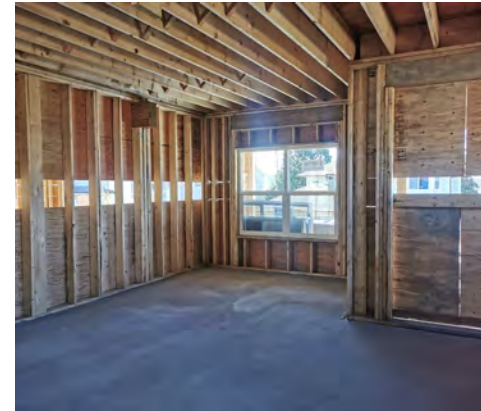
Framing of house (interior)
